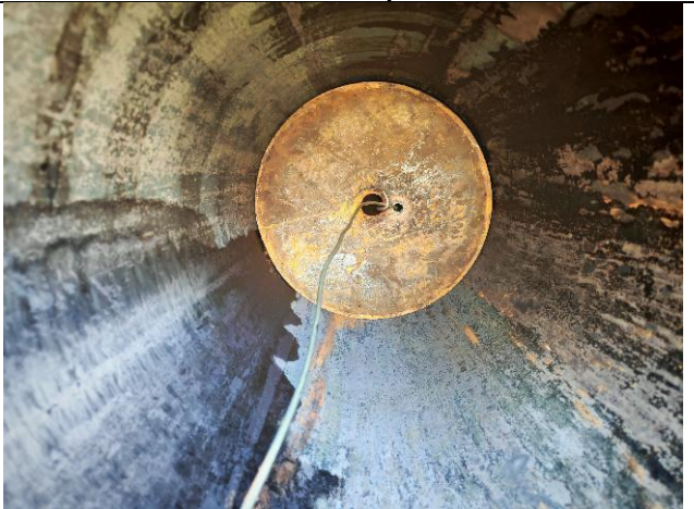
drift test inspection
