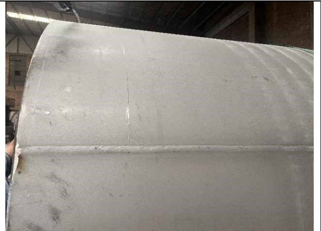
WELD SEAM VISUAL CHECK
